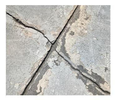
Once all the cracks were cleaned out and the debris carted away, cold patch was placed into the large holes and hot filler was poured into the cracks. Applying the 5 bags of the cold patch and 20 blocks of melted crack filler went like this:
