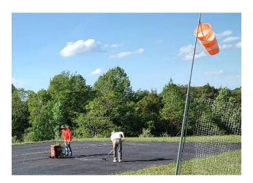
Once the cracks were finally filled, a coating of seal coat was sprayed on the entire runway and taxi way. This was much faster than trying to do it by hand with squeegees:
